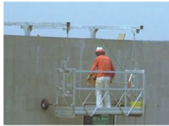
For Wall Plastering
